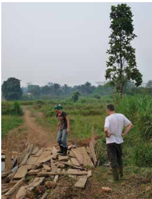
The researchers inspect the bridge on the road to Meliandou.
