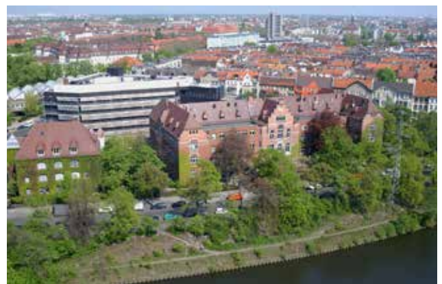
(b) The former laboratory building (silver) accommodating the EM group in Virology on the third level, since 1999 in the basement. The Consulting Lab is an integral part of the EM group Fachgebiet ZBS4. Photo by Andrea Schnartendorff, RKI
